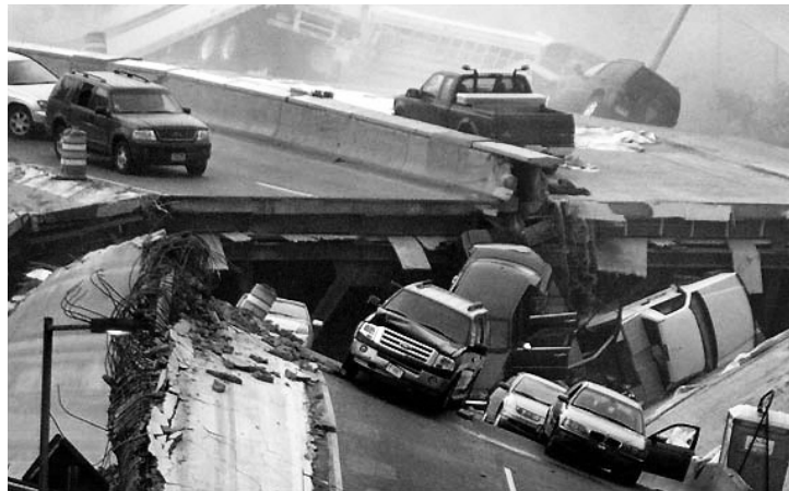
In August 2007, the collapse of the eight-lane bridge in Minneapolis carrying Interstate-35W over the Mississippi River took the lives of 13 people and injured more than 100 others.
