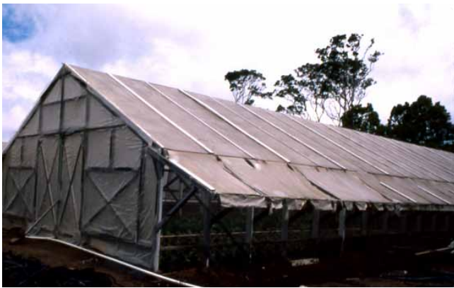
Figure 2. Polyethylene-covered rain shelters with frames (top to bottom) of bamboo (quonset and gable; Sunada Farm, Kainaliu), metal plus lumber (quonset; CTAHR Master Gardeners, Hilo), and lumber (gable with battens; CTAHR Volcano Research Station).
