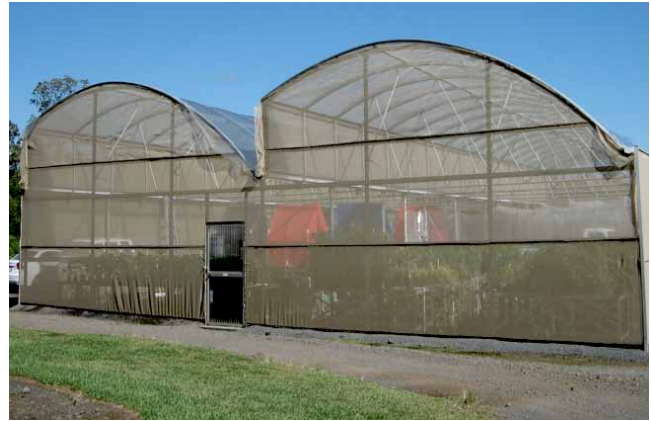
Figure 4. Top-vented (CTAHR Volcano Experiment Station) and upper-side-vented rain shelters (Mel Nishina, Hilo).
