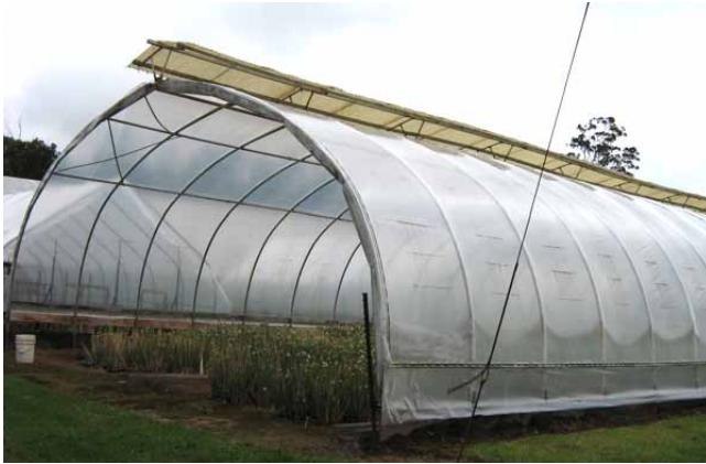
Figure 4. Top-vented (CTAHR Volcano Experiment Station) and upper-side-vented rain shelters (Mel Nishina, Hilo).
